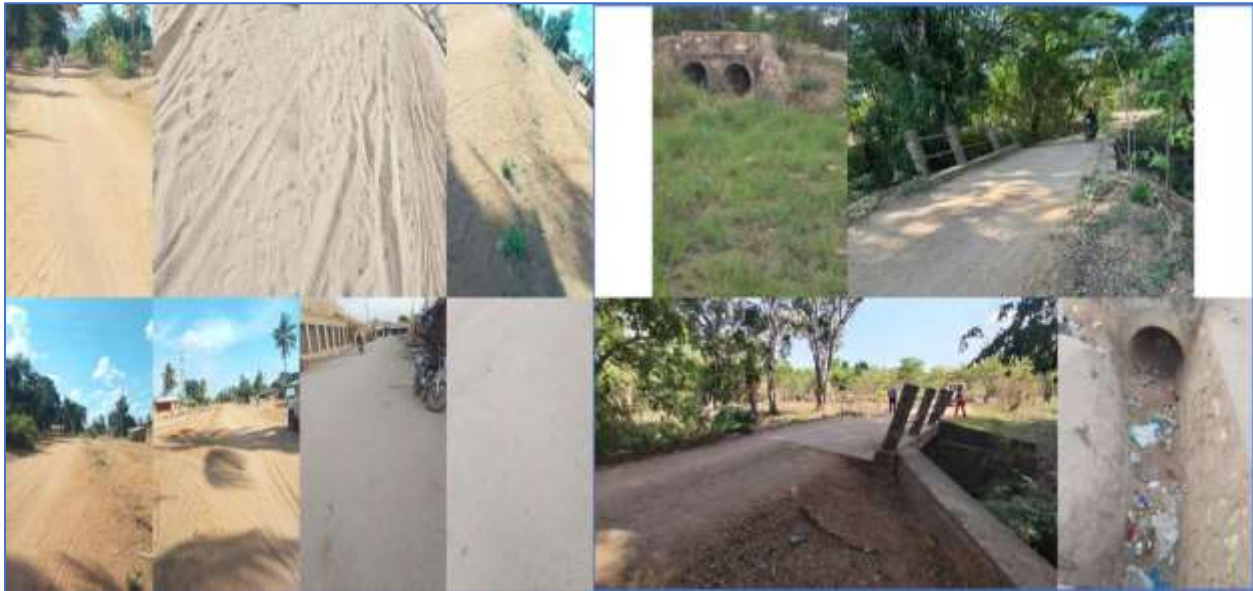
Figure 13: Observed Bridges and Culverts
